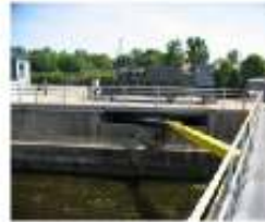
Picture 45: Mitre Gate Drive – Modified Ohio Linkage United States Army Corps of Engineers
