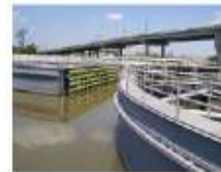
Picture 46: Sector gate New Orleans District United States Army Corps of Engineers – Drive gear on front face of sector gate
