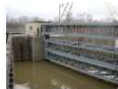
Figure 78. GM River Lock New Orleans District United States Army Corps of Engineers - These emergency bullheads are designed to be set under differential head and flowing water and are also utilized in maintenance bullheads.
