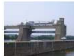
Figure 74. Bullhead Crane with Auxiliary "Frigidlock Crane" at Racine Dam on the Ohio River. One Bullhead Section is Stored in each Gate Bay.
